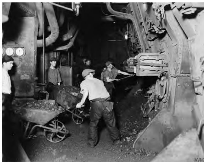
Steam ships boiler room
